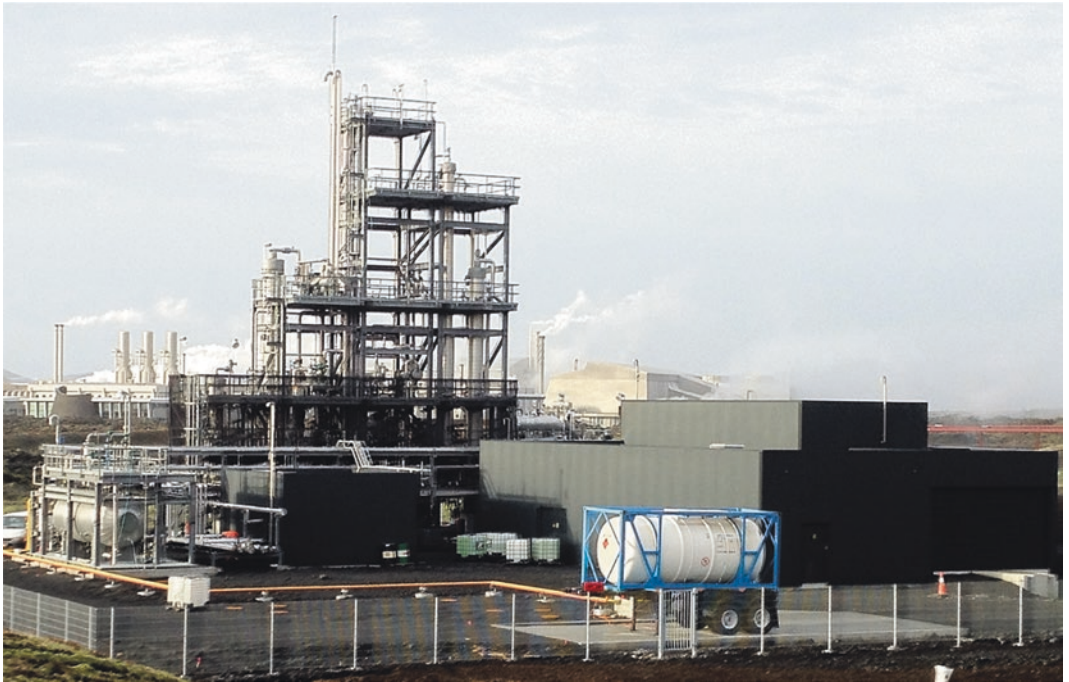
▣ Abb. 14.20 Die Methanolanlage »George Olah carbon dioxide to renewable methanol plant« der Carbon Recycling International in Grindavik, Island (Quelle: CRI)
